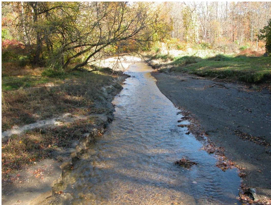
Photograph 4. Above the dam looking upstream with water level boards removed and pond drained, showing the degradation of the natural channel and silt buildup
