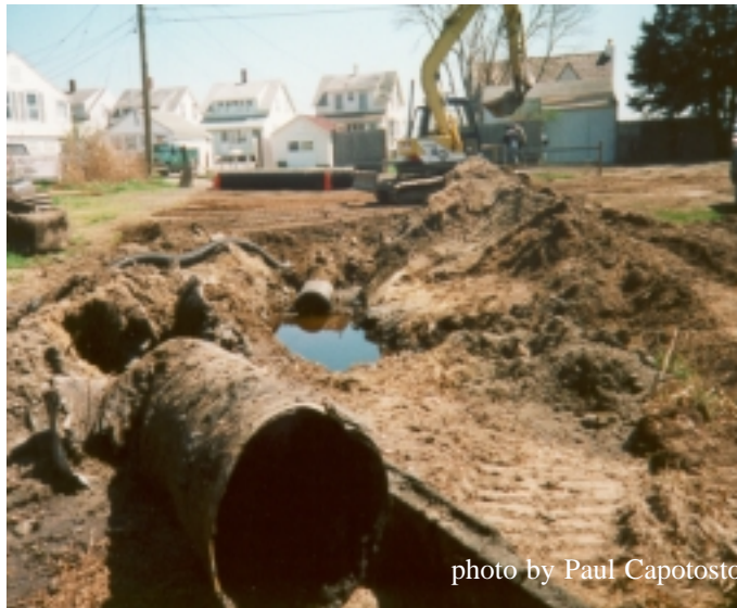
Replacement of an 18” pipe with a 24” pipe for allowing natural flow into the marsh
