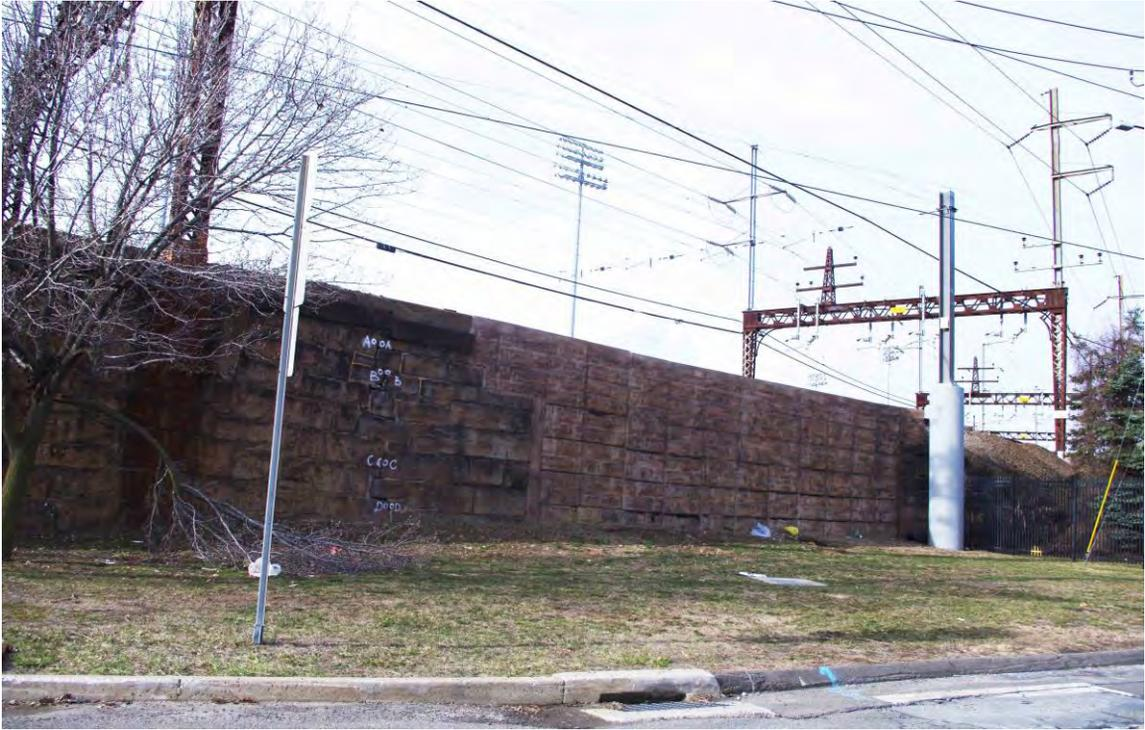
**Photograph 65. Infilled section of the railroad viaduct where the Main Street Bridge was removed, camera facing northeast.**
